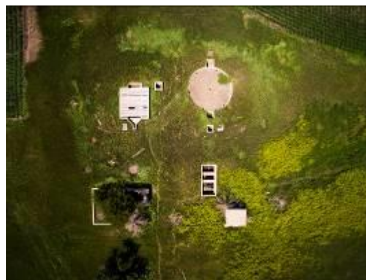
Abandoned Sewage Treatment Plant – Aerial View
