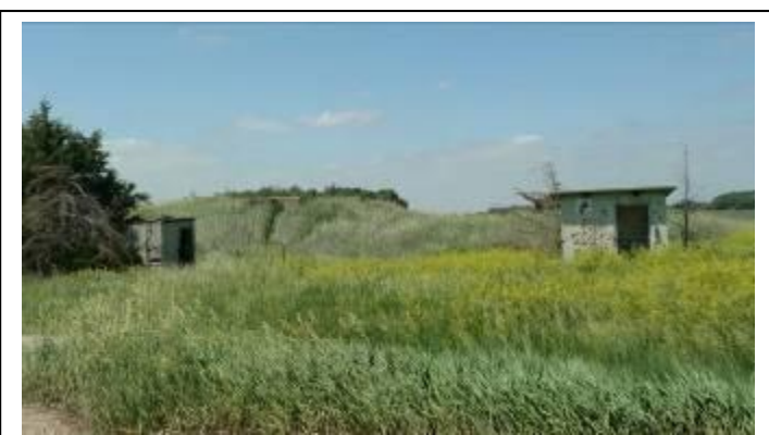
Abandoned Sewage Treatment Plant
