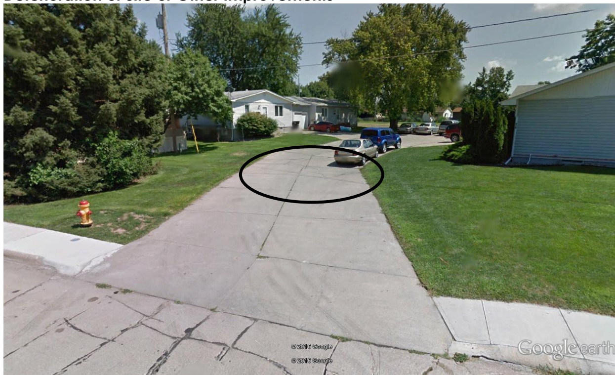
Figure 5 Deterioration of Site or Other Improvements
