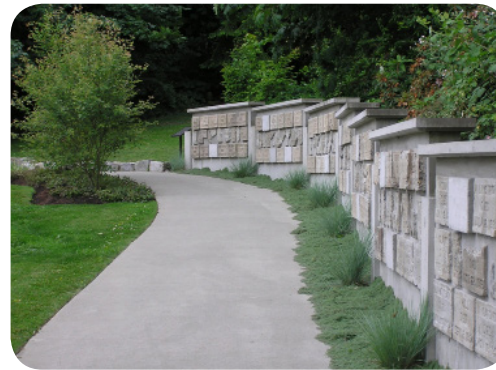
Wall along Path
