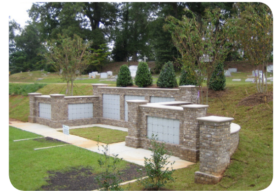
Retaining wall 'room'
