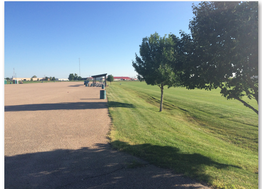
Edge of a asphalt parking lot gives way to a drainage swale.
