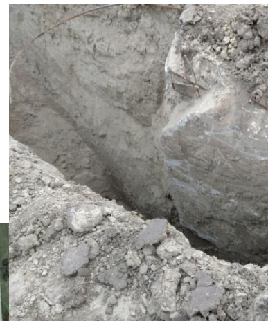
A recently unearthed concrete footing on the site.
